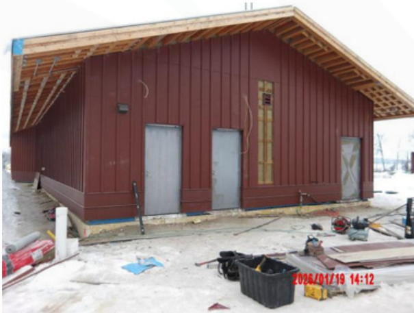
Siding installs for one of the detox buildings
