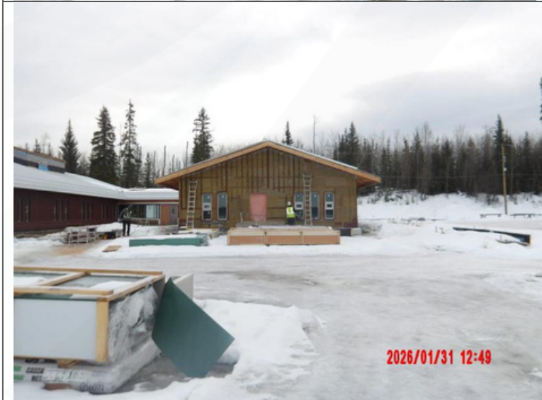
Strapping of the admin building
