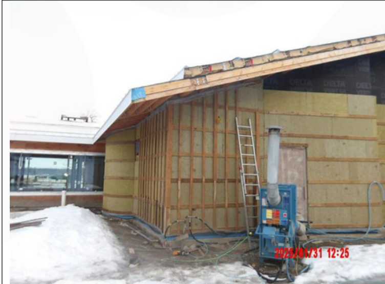
Strapping on one of the residential therapy buildings
