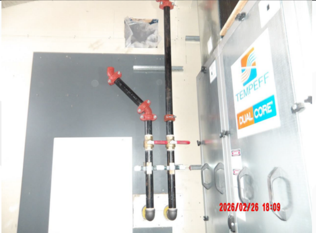
Plumbing rough in, West residence penthouse
